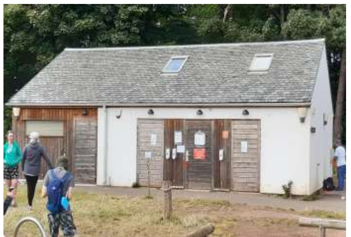
Photo 8. Toilets, Yellowcraigs, East Lothian
